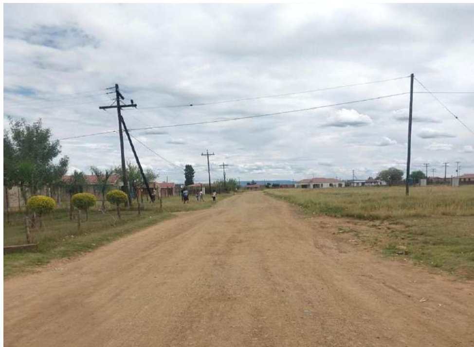
Figure 3: View of some power lines traversing through the project area in the Ndongwane area.
