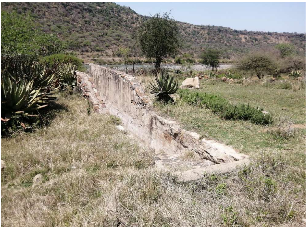
Figure 30: Showing the derelict dip tank identified on site MHB01 .
