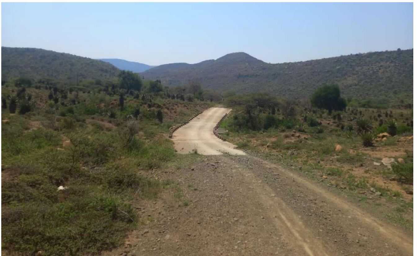
Figure 14: Showing existing access roads within the study area.
