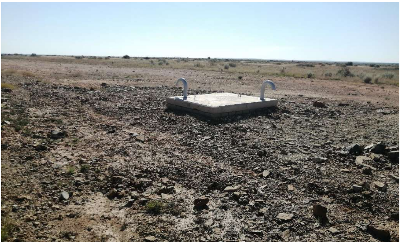
Figure 7: Showing bulk water infrastructure, proposed development site is heavily disturbed.
