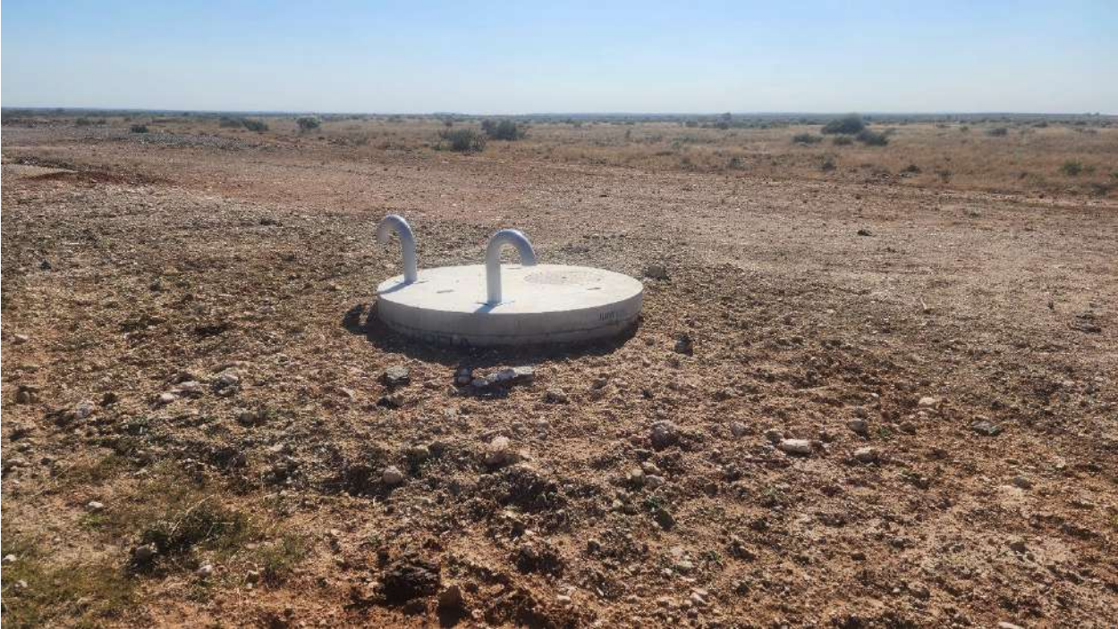
Figure 7: Underground pipeline constructed on site
