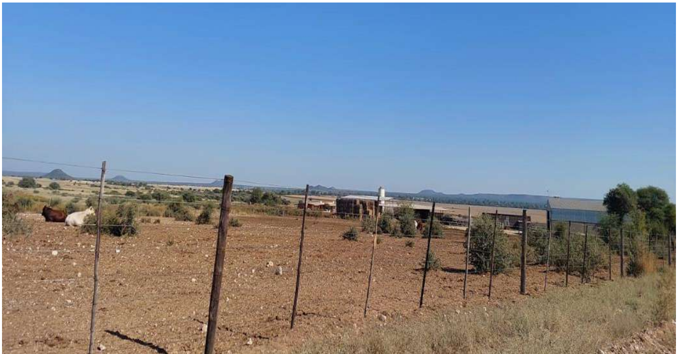
Figure 26: Showing the farm structures in the background.
