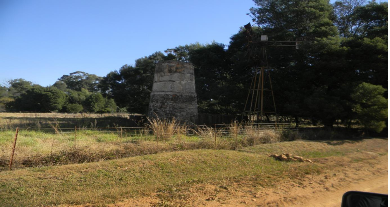
Plate 21: showing farm structures that are likely to be over 60 years
